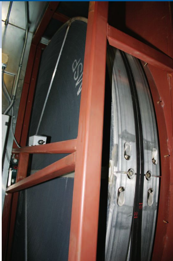
This “enthalpy wheel”—located in building E62—preconditions incoming air so as to reduce the need for heating and air conditioning. The wheel salvages useful energy from used building air and transfers it to incoming fresh air, warming and humidifying it in the winter and cooling and drying it in the summer.
