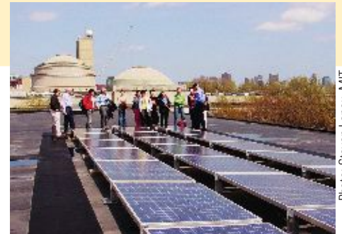
These solar panels on the roof of the Student Center were among the MIT installations examined by students in Fundamentals of Photovoltaics. By analyzing years of energy output data, the student team detected unexpected losses of efficiency, thereby identifying steps that MIT can take to improve PV performance.
