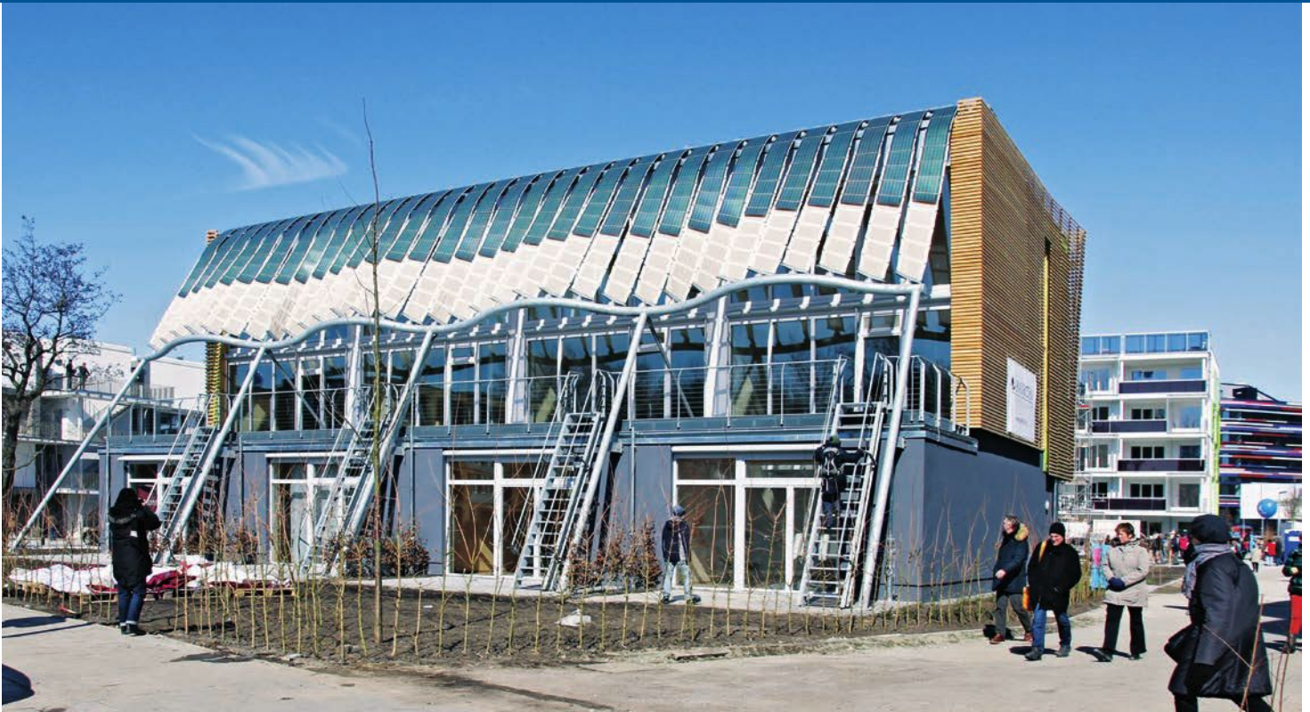
The Soft House, an innovative work/live row housing project, is now demonstrating novel concepts in energy and architecture at the IBA in Hamburg, Germany. The four housing units include a responsive energy-harvesting textile façade and movable light-emitting interior curtains that enable occupants to reconfigure their domestic space, creating a flexible new model for carbon-sequestering architecture. Each unit has a terrace space, a PV canopy, and a vertical convection atrium layer that circulates air, brings daylight into the ground floor, and creates vertical views of the sky.
