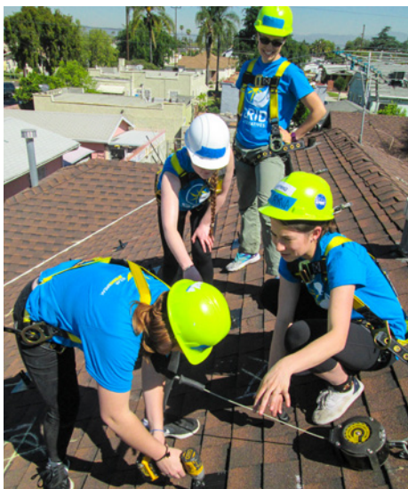
Left: Secured to the roof by harnesses, the students install “flashings”—black mounts that serve as foundations for the solar panel installations.
