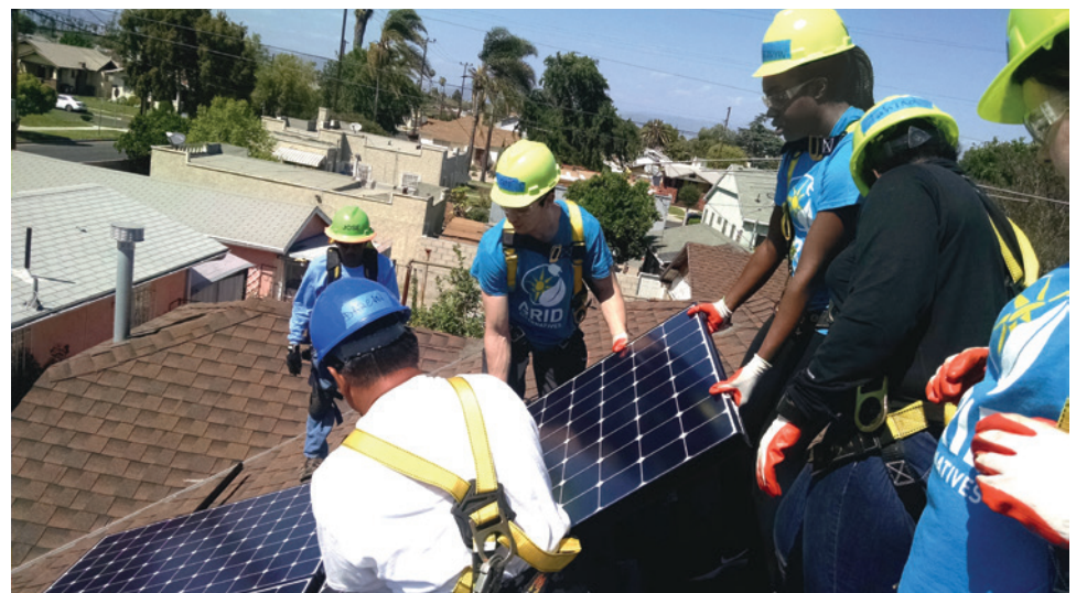
Left: Secured to the roof by harnesses, the students install “flashings”—black mounts that serve as foundations for the solar panel installations.
