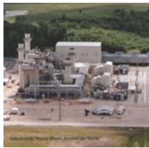
Natural-Gas Combined Cycle
