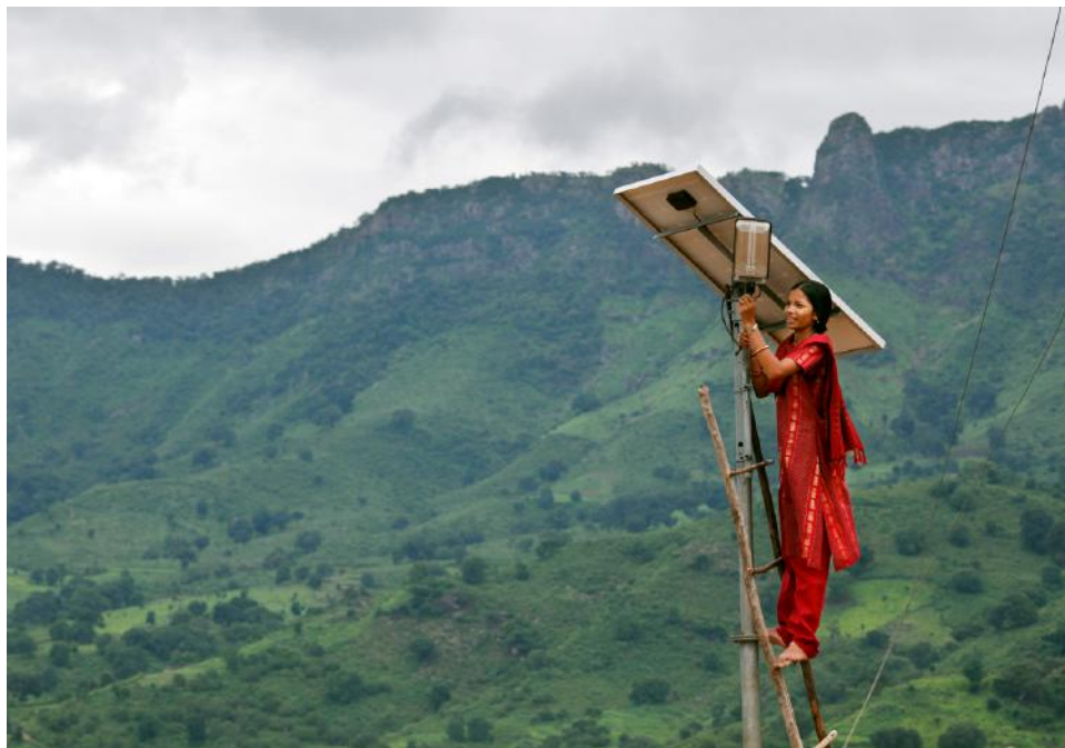
A solar engineer maintains the street lighting in her village of Tinginaput, India—a rural area not connected to the region's main electrical grid. Photo: Abbie Trayler-Smith/Panos Pictures/Climate Visuals
