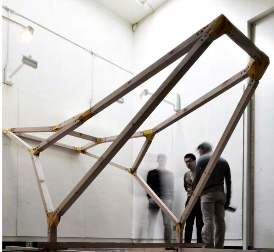
The researchers produced and installed this structure on the MIT campus using waste tree forks as structural elements. In the future, they plan to use their process to design and build a complete outdoor pavilion, which will be located at the site of the felled trees from which the wood forks were recovered. Photo: Felix Amtsberg
